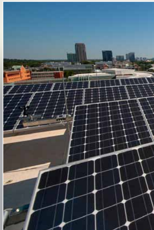
The solar panels atop the new Clough Undergraduate Learning Commons help make the facility one of the most sustainable on any university campus.
